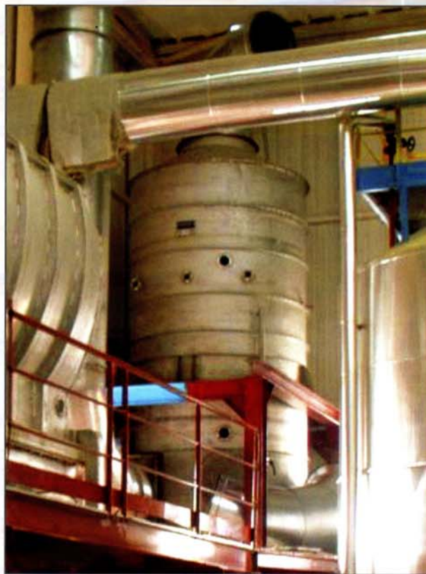
Wet swirl scrubber installed in the sugar Factory Kruszwica S.A., capacity 18m 3 /s, made of stainless steel.
