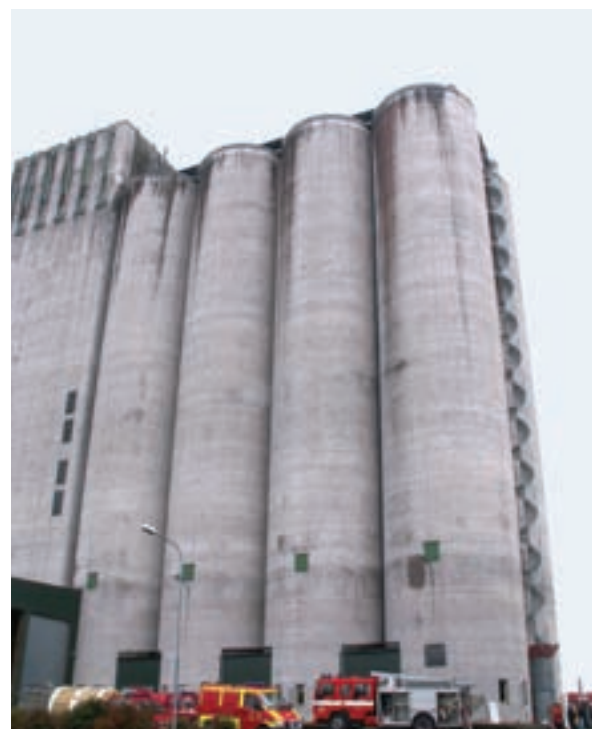
Figure 5: the silo on fire (second from right) was 47m high, 8 m in diameter, and filled to about 40m with wood pellets. A vaporisation unit was used to ensure that the gas was injected in gaseous phase.
