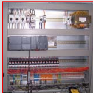
Control of a water treatment plant with caustic soda at Thyssen-Krupp in Andernach, Germany.
